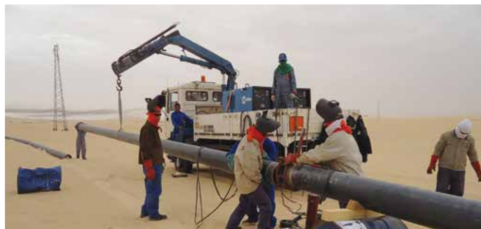
10" Trunk Line at 5J Area Waha Oilfield Project
